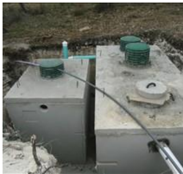
Figure 5. Biological Accelerated Treatment plant during installation
