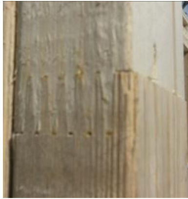
Figure 4. Finger-jointed stud used in the residence construction
