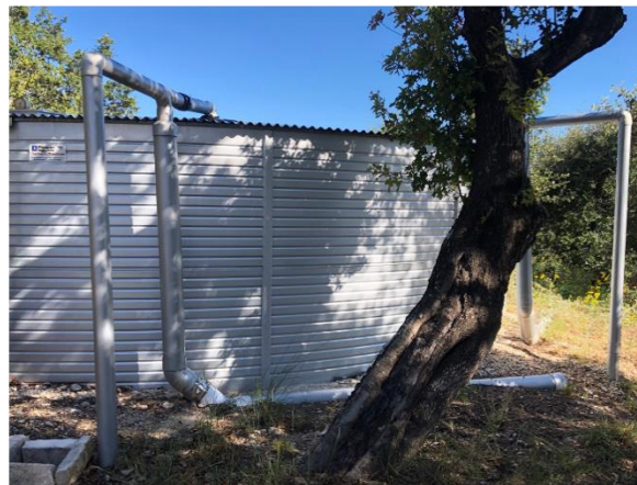
Figure 8. First flush system
