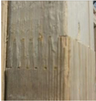
Figure 4. Finger-jointed stud used in the residence construction
