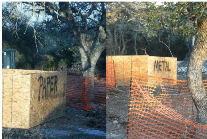
Figure 3. Bins established for paper / metal collection during construction
