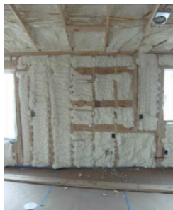
Figure 3. Open-cell spray-foam insulation installed in the residence
