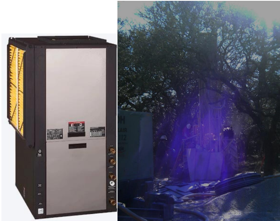
Figure 22. Geothermal unit and vertical drilling of wells
