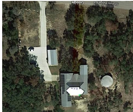
Figure 1. The residence as constructed
