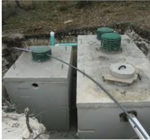
Figure 16. Biological Accelerated Treatment plant during installation
