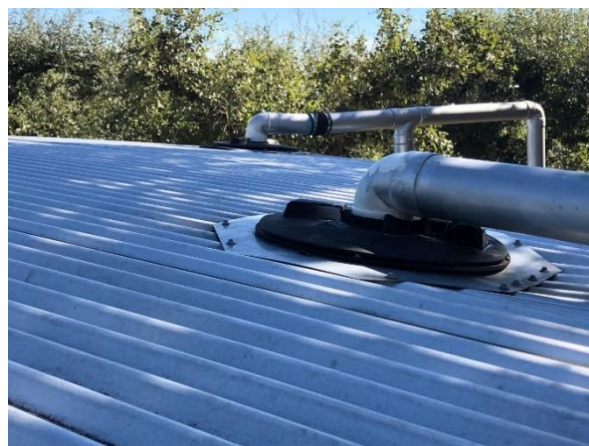
Figure 8. First flush system
