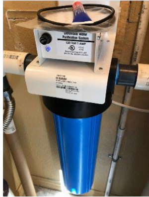
Figure 13. Ultraviolet purification and example light
