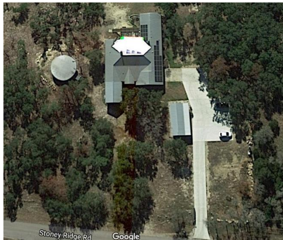
Figure 1. The residence as constructed
