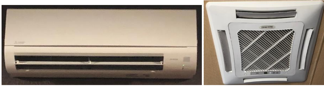
Figure 20. Mini-split units, in wall and in roof
