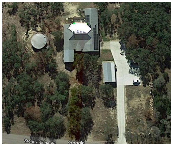
Figure 1. The residence as constructed
