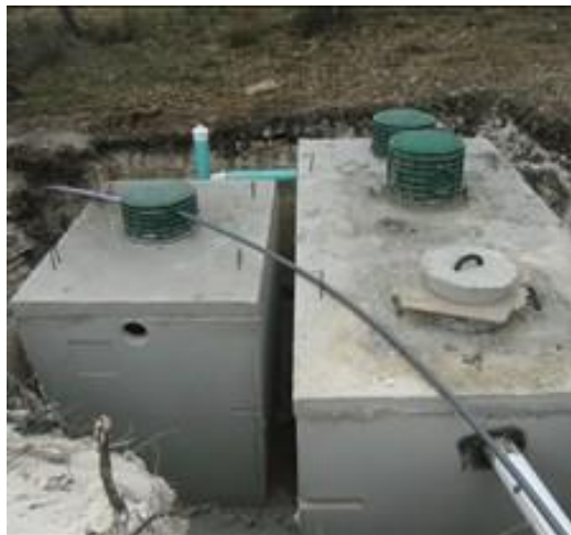
Figure 14. Biological Accelerated Treatment plant during installation
