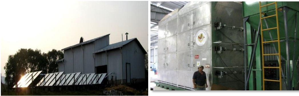
Figure 3: The Off-Grid Facility- the first Solar Power based industrial plant
